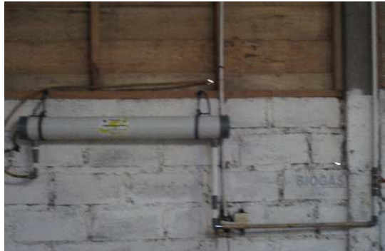
Gambar 4. Instalasi Filter Biogas
